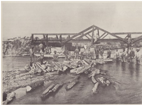
Figure 2: The original Cradlebaugh Bridge
